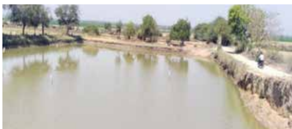
De-silted water harvesting structure in the watershed
