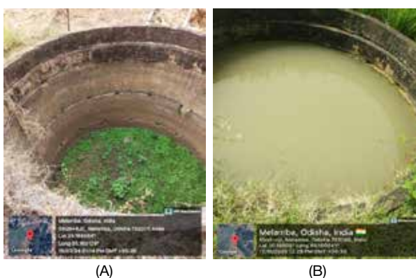
(A) Depth of water table before (A) and after (B) construction of the recharge shaft in the dugwell located in the Melamba village, Nayagarh, Odisha
