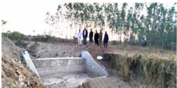
Repair of inlet and outlets of the water harvesting structure
